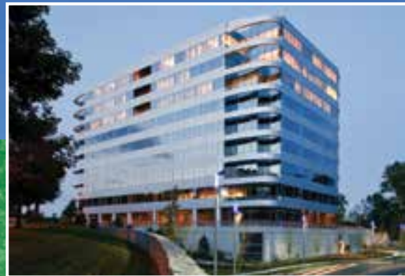
2000 Tower Oaks Blvd LEED Platinum
